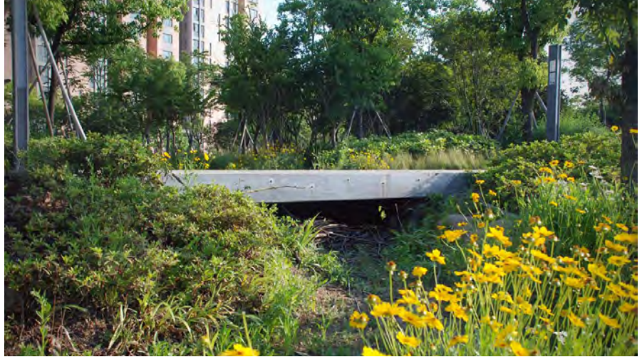
Example of bridge over vegetated swale
