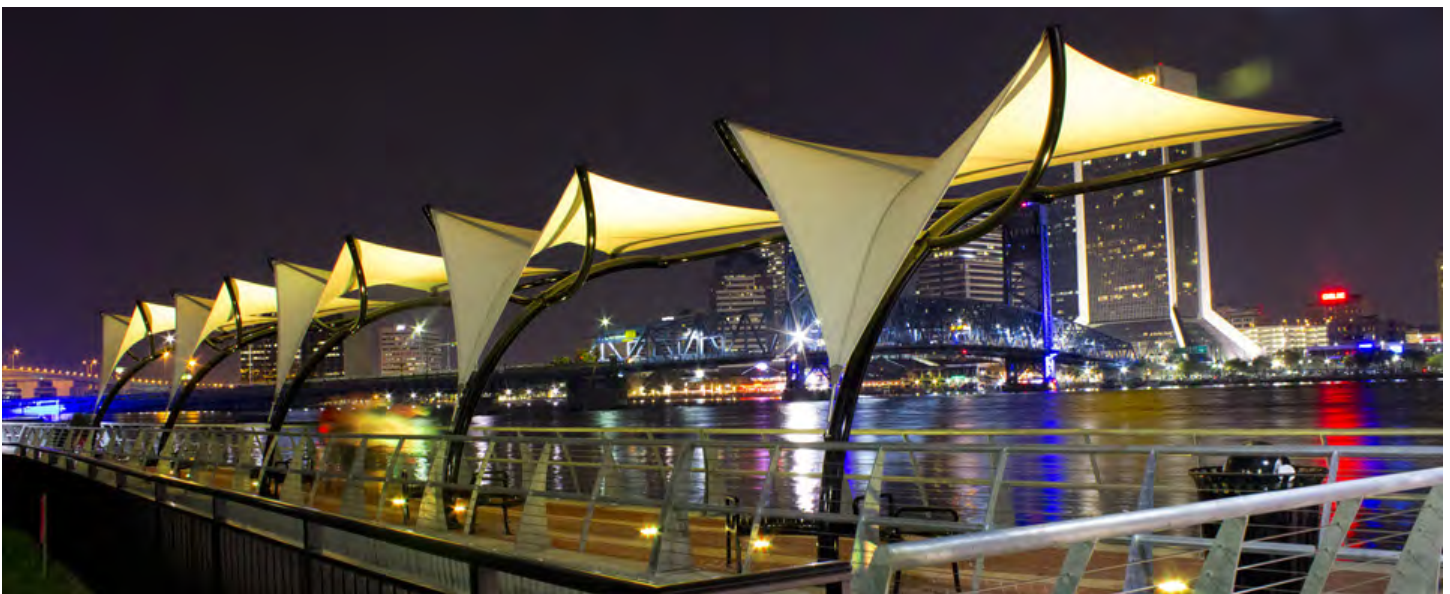
Photo: Shade Systems
