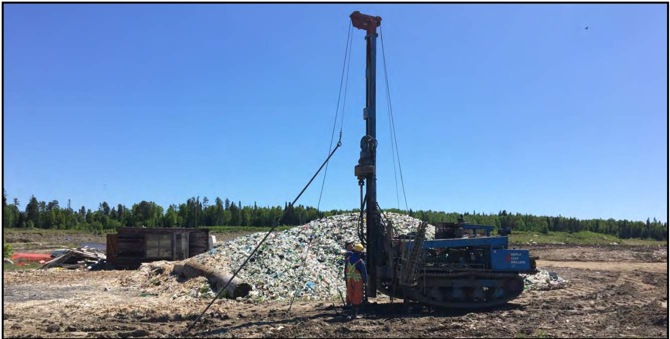
PHOTOGRAPH #4: View of TH2 during drilling as seen facing south.
